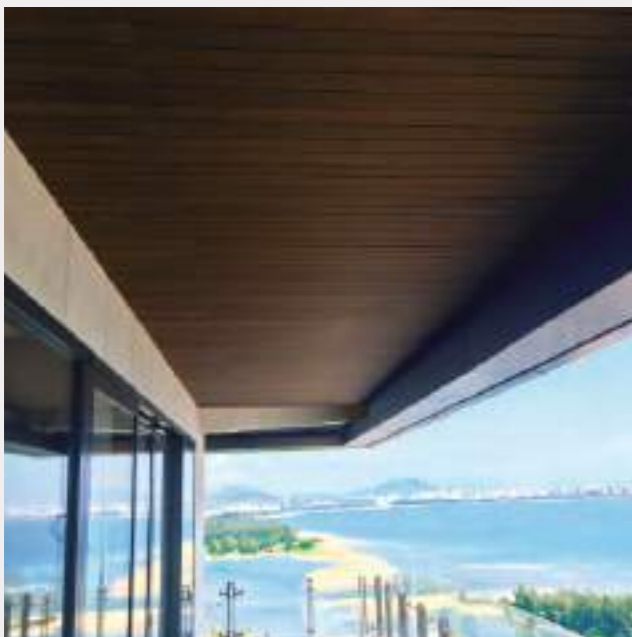
Soffit Easy hidden fastener system Structural T&G end match
