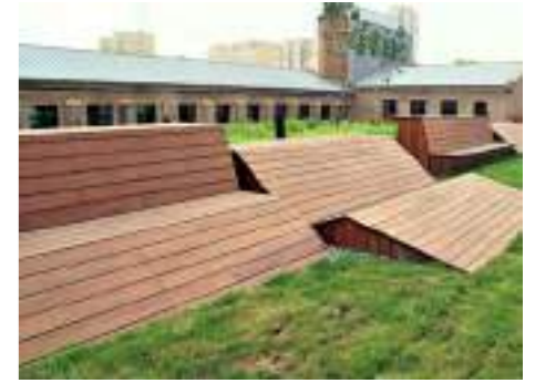
Reconstruction of Jilin Waterworks
